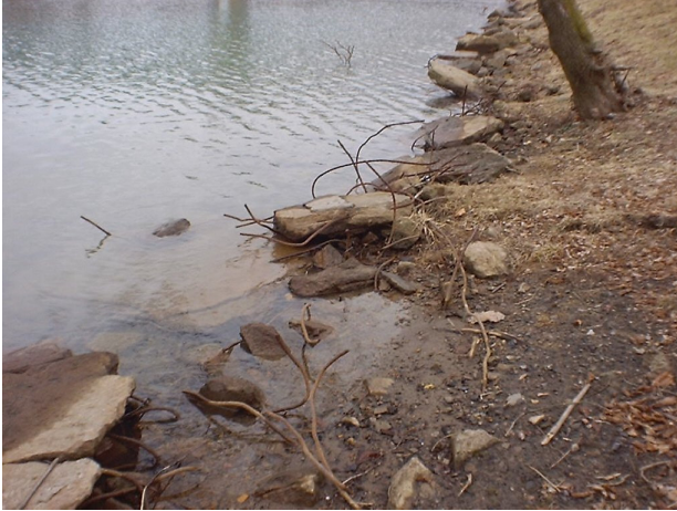
Hazardous condition at McQuain Park
